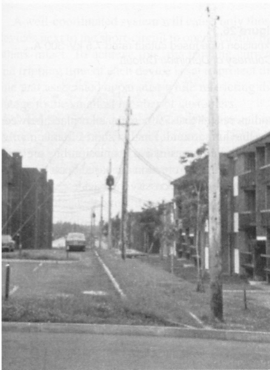
Figure 26.28 MV aerial feeder serving a residential district.
